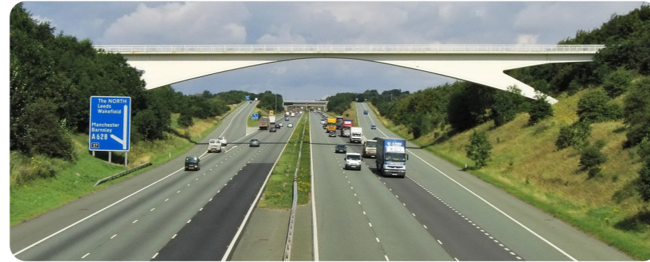
M1 motorway in Yorkshire
